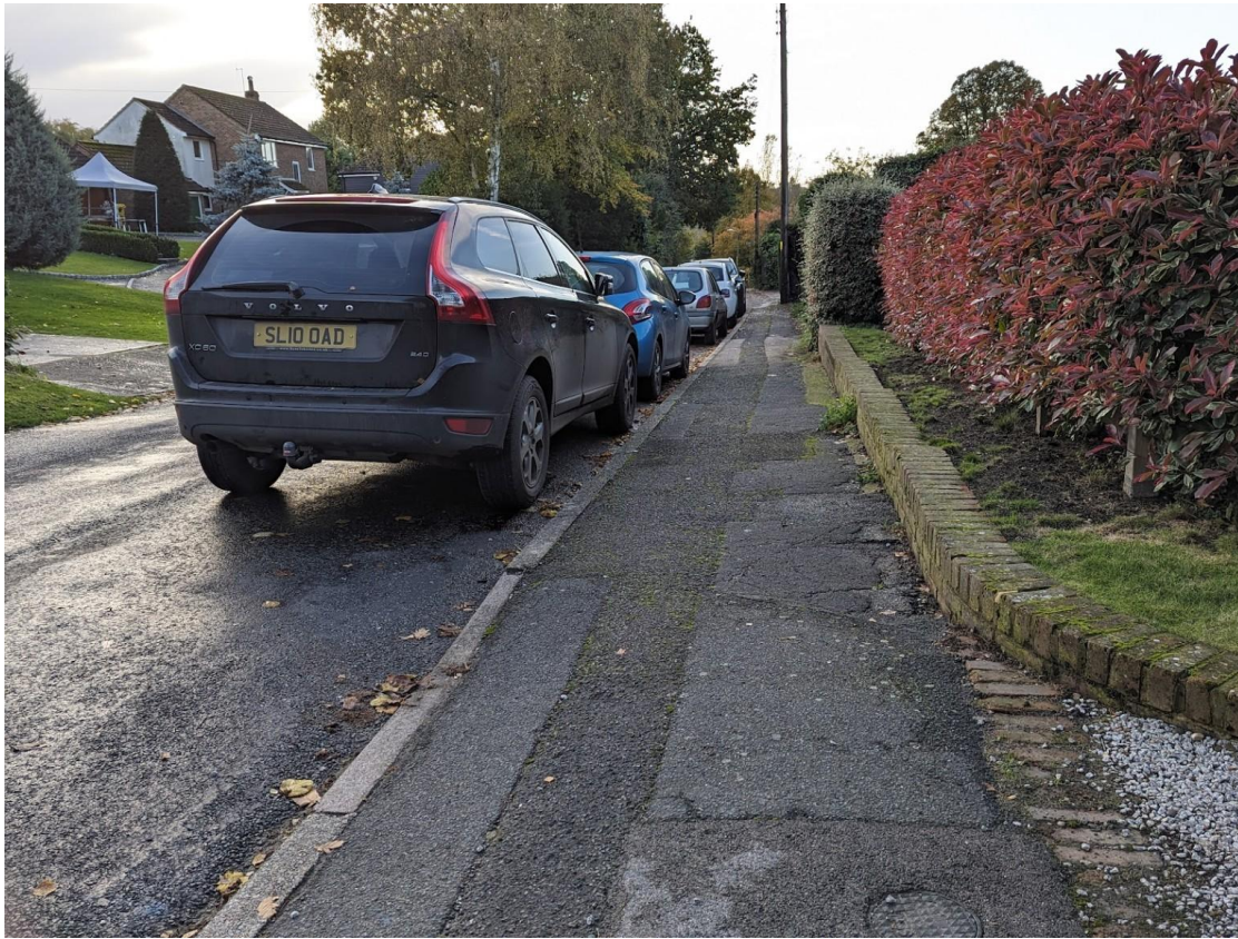
Figure 4. Parked vehicles directly adjoin a narrow and uneven footway.
