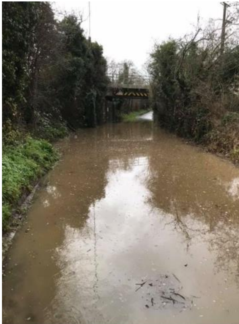
Figure 2 – Fox Lane Bridge, December 2020
